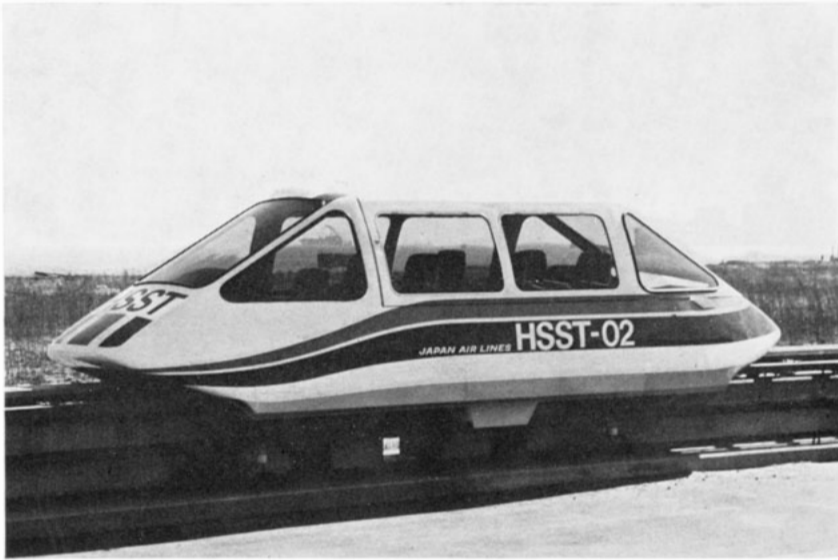
Figure 9. Japan Air Lines 8 passenger vehicle HSST-02. (Reproduced by permission of Japan Air Lines.)
